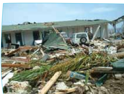
Damage from Tropical Cyclone Heta, January 2004.
